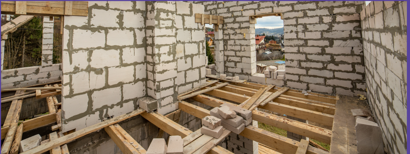
Image: Building site of a house under construction made from white foam concrete blocks. Source: original image by Africa images
